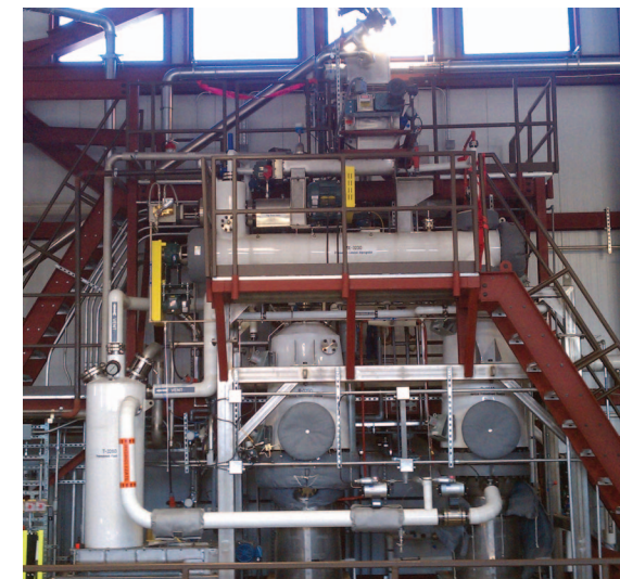
Photo by Dennis Schroeder, NREL/PIX 19527
