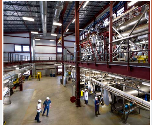
NREL's biochemical conversion pilot plant is located in the Integrated Biorefinery Research Facility (IBRF). Photo by Dennis Schroeder, NREL/PIX 20248
