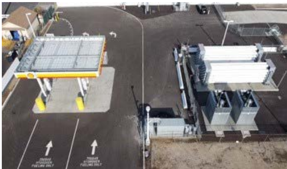
Figure 26. Aerial Photo of the Wilmington Station
