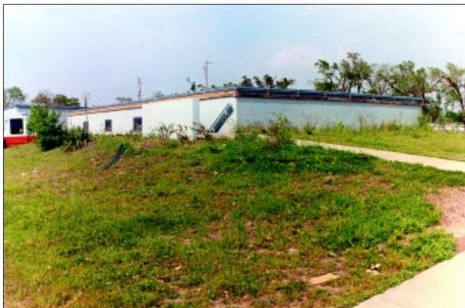
FIGURE 6-9: Partially belowground community shelter in a manufactured home park in Wichita, Kansas.
