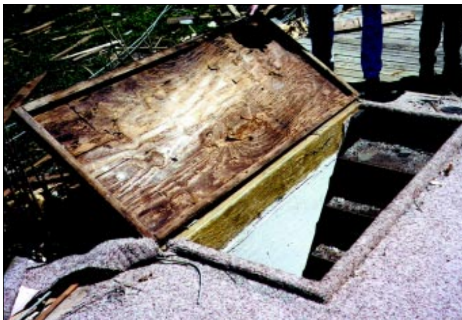
FIGURE 3-31: Underground residential shelter, viewing door and stairway leading down to shelter. This shelter was located outside a residence.
