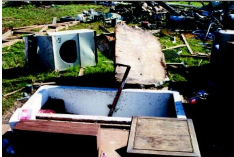
FIGURE 6-12: Failed wooden door at a belowground shelter in Oklahoma. Note the medium-size debris (clothes dryer) immediately adjacent to the shelter access.
