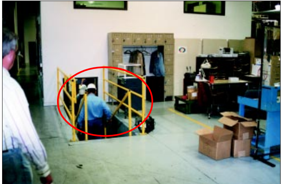
FIGURE 6-7: Entrance to the plastics manufacturing plant group shelter in Haysville, Kansas.
