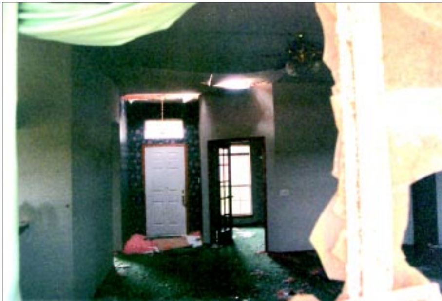
FIGURE 4-30: View of interior of the home shown in Figures 4-28 and 4-29.
