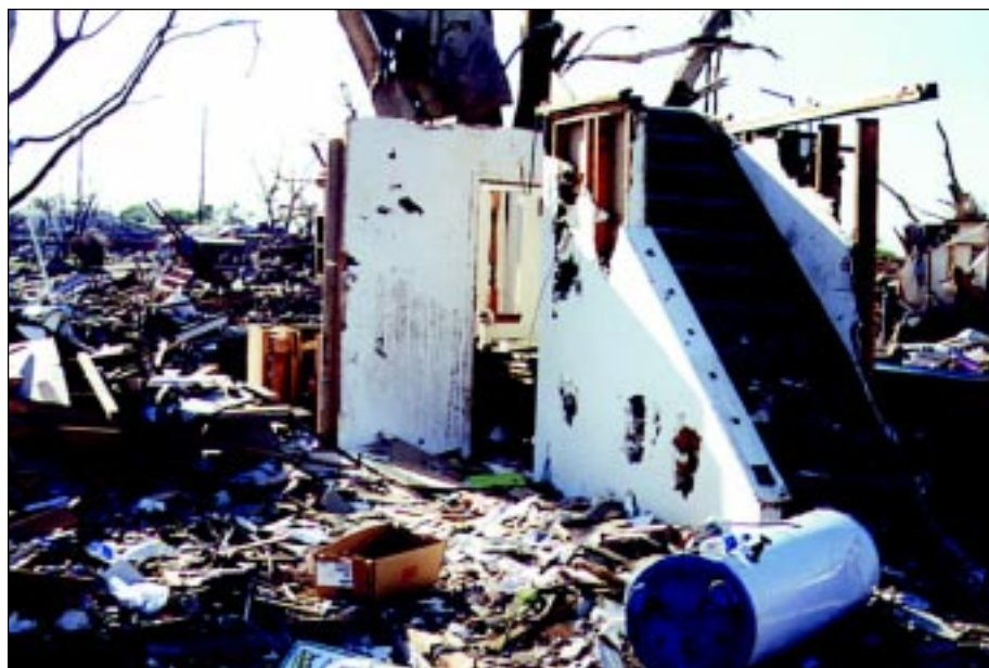
FIGURE 6-31: The core remnant of this house was beneath the staircase to the second floor.
