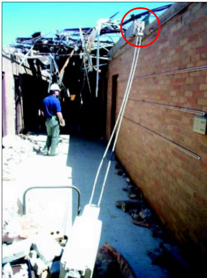
FIGURE 5-3: Kelly Elementary School, in Moore, Oklahoma, hit by vortex of violent tornado. Damage to school displaying separation between the bond beam and supporting wall and separation between bond beam and roof bar joists.
