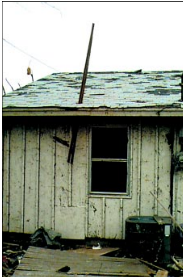
FIGURE 3-18: This missile fell nearly vertical, illustrating the importance of a strong cover over the top of a tornado shelter to protect against free-falling debris. This home was located in Midwest City,
