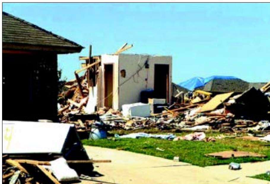
FIGURE 6-28: The core remnant of this house consisted of a central room and closets.
