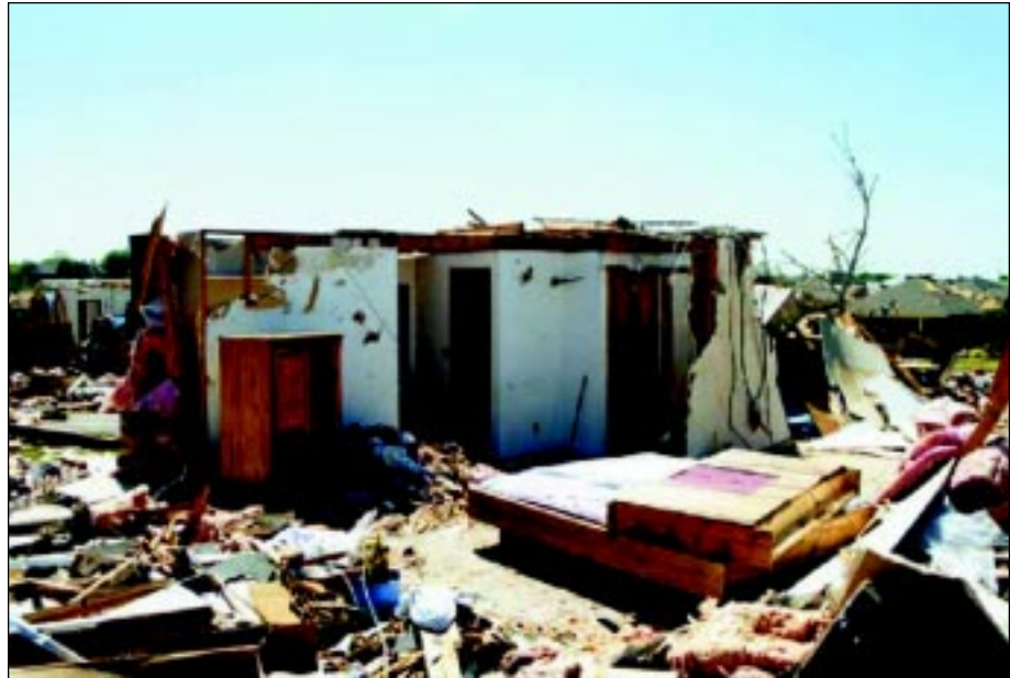
FIGURE 6-29: The core remnant of this house consisted of a central room and adjacent closets.
