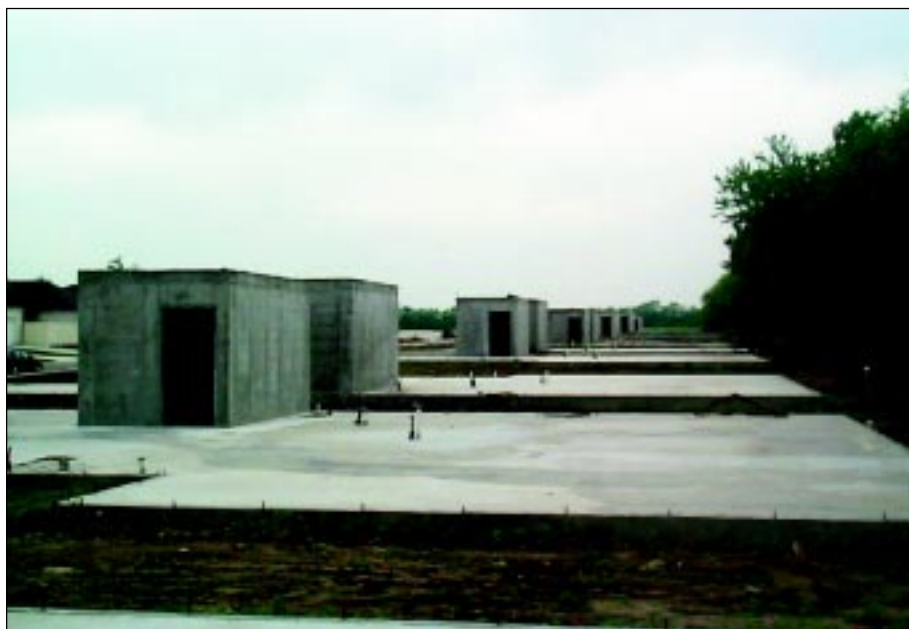
FIGURE 6-6: Aboveground in-residence shelters under construction in Wichita, Kansas.
