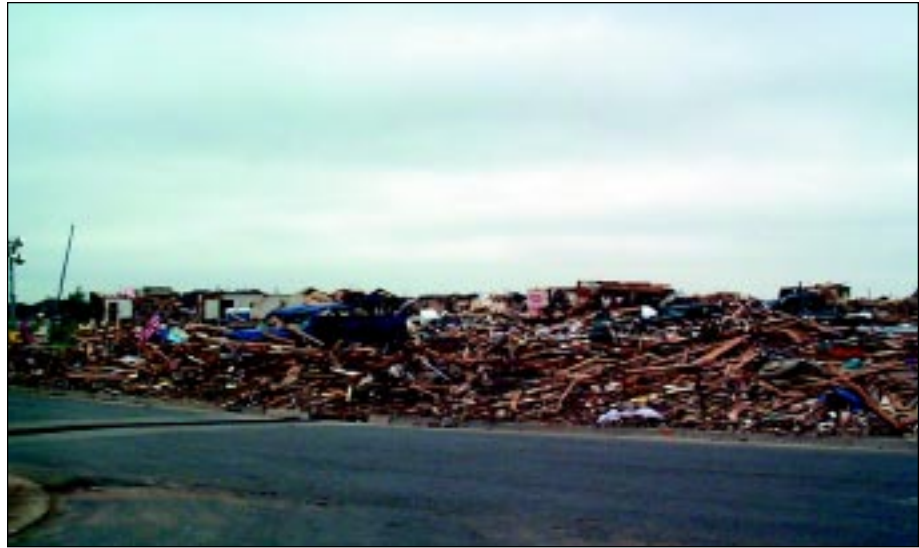
FIGURE 3-26: Debris generated by the vortex of a violent tornado in Moore, Oklahoma, created a layer of rubble across the ground.
