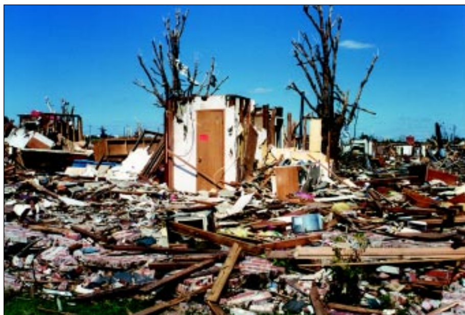
FIGURE 6-19: Remains of an interior room (or core) of a home in a Moore, Oklahoma, subdivision that was hit by a violent tornado.
