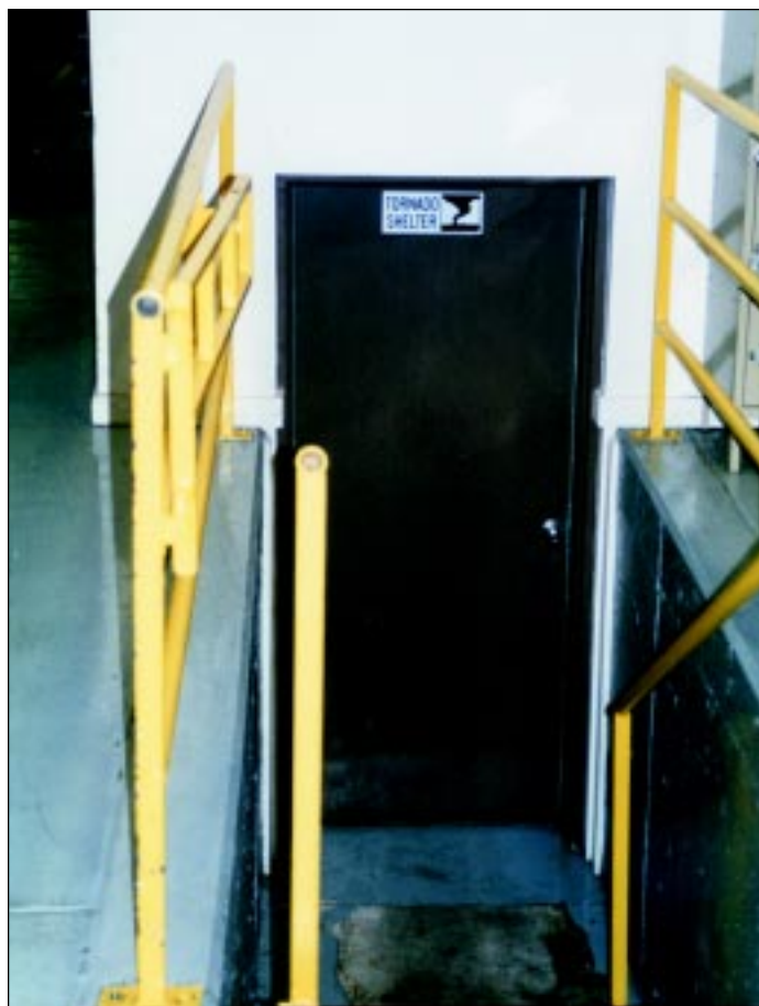
FIGURE 8-12: Example of a tornado shelter provided in a place of business in Haysville, Kansas.
