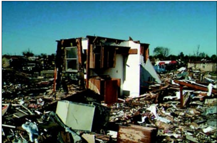
FIGURE 6-30: The core remnant of this house was a central room on the back of the kitchen.
