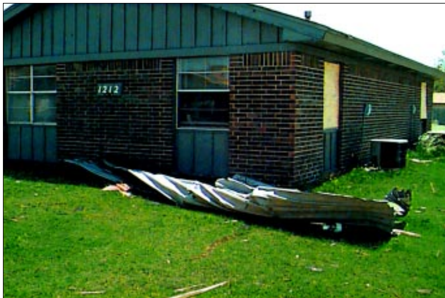
FIGURE 3-21: This piece of steel deck landed at the periphery of a violent tornado damage area in Moore, Oklahoma. The building it likely came off of was a few hundred feet away.
