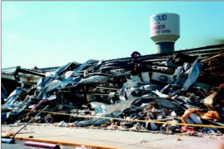
FIGURE 5-9: Stroud Regional Outlet Mall, Stroud, Oklahoma, was struck by the vortex of a weak tornado.
