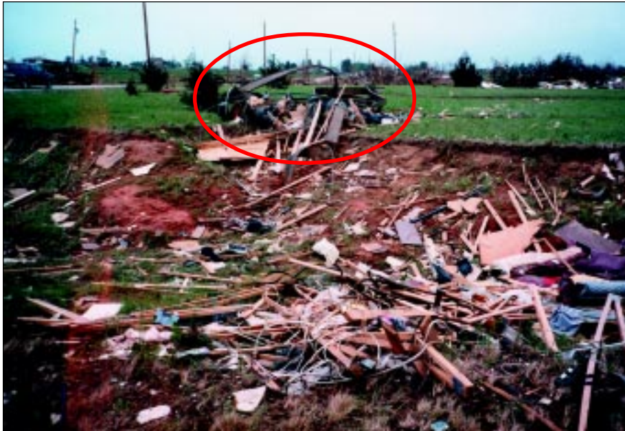
FIGURE 4-47: This 14-ft x 60-ft manufactured home chassis in the background of this photo moved about 200 yards from its original anchoring site in Figure 4-49, Bridge Creek, Oklahoma.
