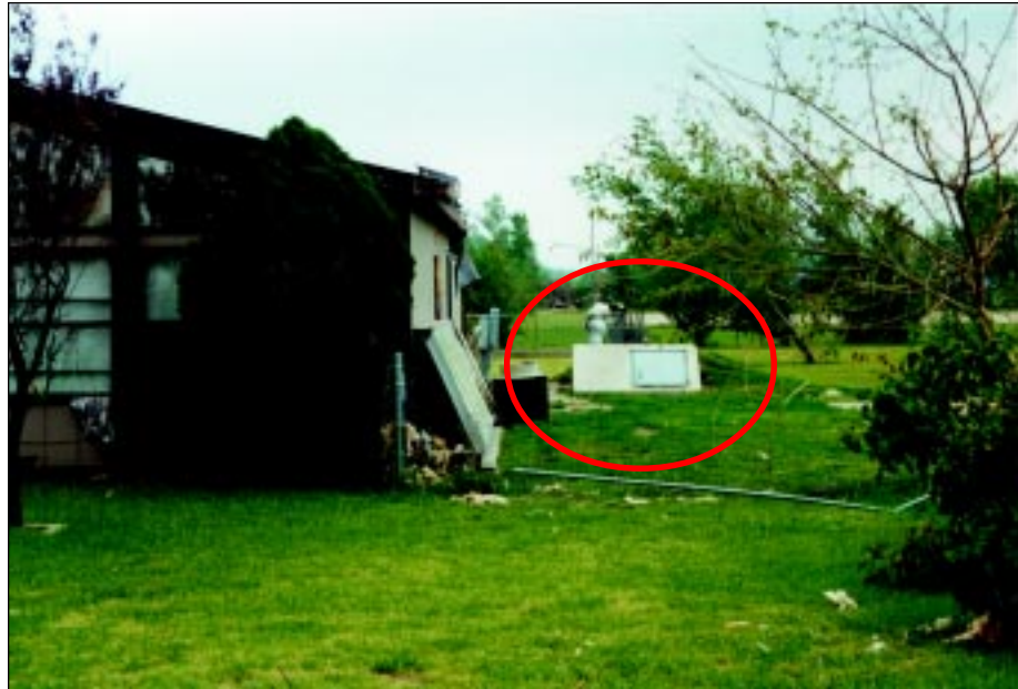
FIGURE 6-4: This precast concrete storm cellar was located immediately behind a single-family residence in Sedgwick County, Kansas. This residence and shelter were on the periphery of a violent tornado path.
