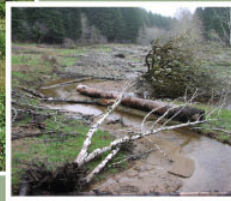
Figure 8. Placing large wood in the Anderson Creek channel and floodplain.
