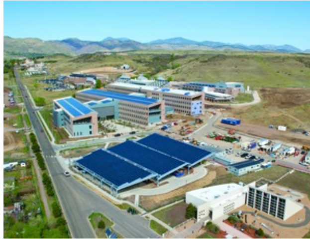
National Renewable Energy Laboratory
