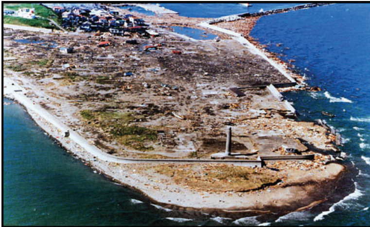
Figure 1-2: A tsunami generated on 12 July 1993 by a magnitude 7.8 earthquake off Aonae, Okushiri Island, Japan, completely denuded the exposed Aonae peninsula of built structures and caused severe damage to the port facilities. Maximum wave height and current speed were estimated to be approximately 10 m and 18 m/s, respectively.
