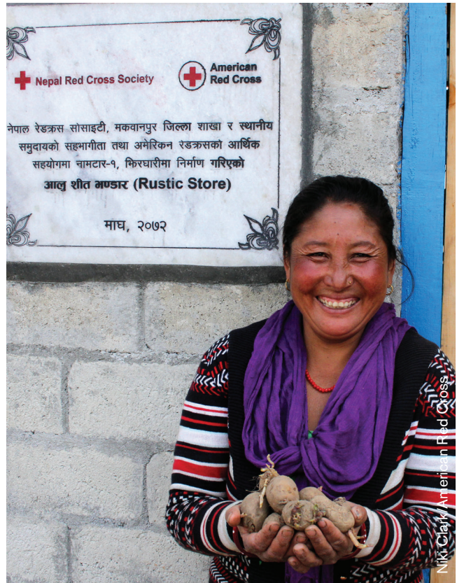
Bisnu Maya Rumba stands outside a new seed potato storage building in Jhir Gari, Nepal, funded by the Red Cross. Bisnu and her neighbors contributed labor, while the American Red Cross and Nepal Red Cross supplied materials, money and technical assistance.
