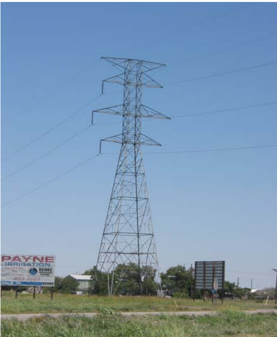
ETL: Metal Truss Tower
