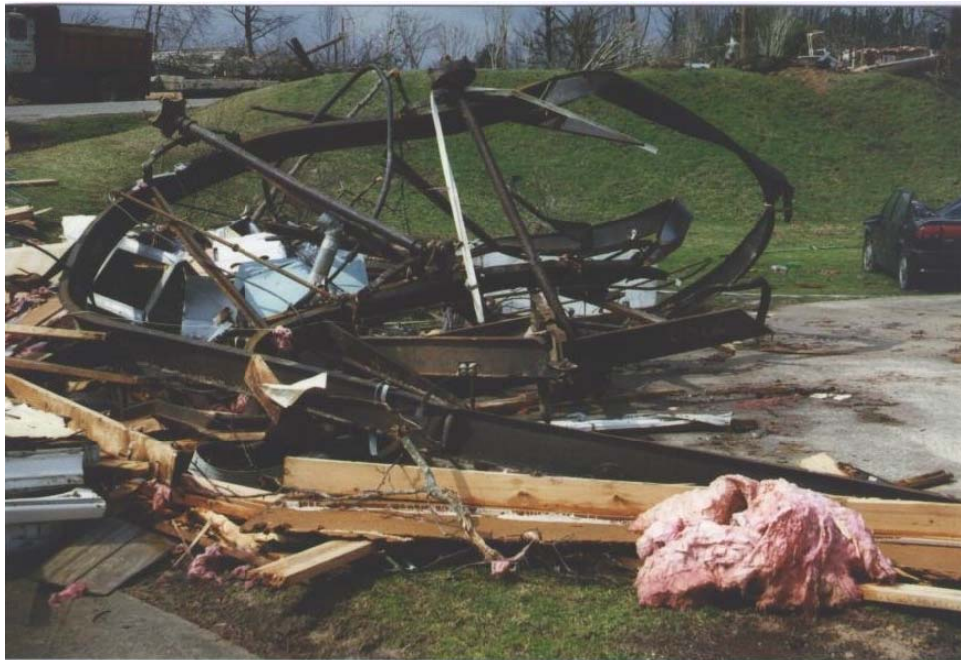
MHDW: DOD 11: Undercarriage separates from floor; rolls and tumbles, badly bent
