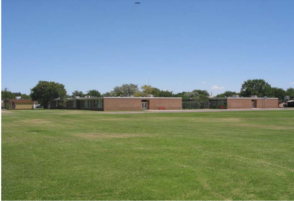
ES: Single story with flat roof; built-up roofing with gravel; brick veneer; large percentage of window glass; long interior hallways; load-bearing walls
