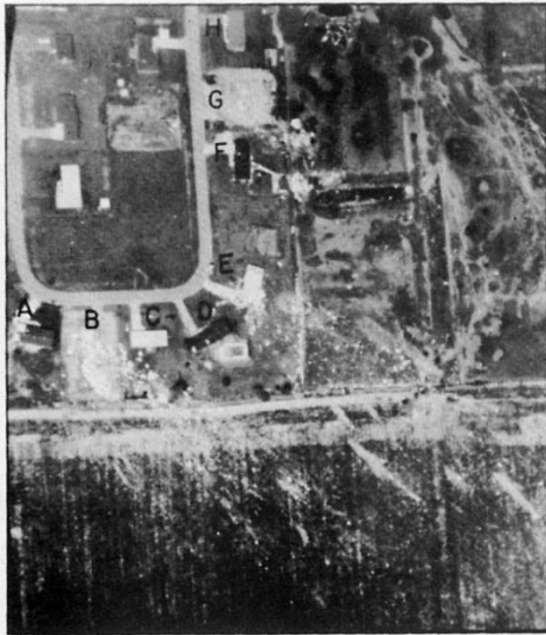
FIG. 20. An aerial view of houses A-H in Fig. 13. Pieces of the roofs were blown into the cornfield, smashing the cornstalks which were about 4 ft tall. Houses B and G were under construction.
