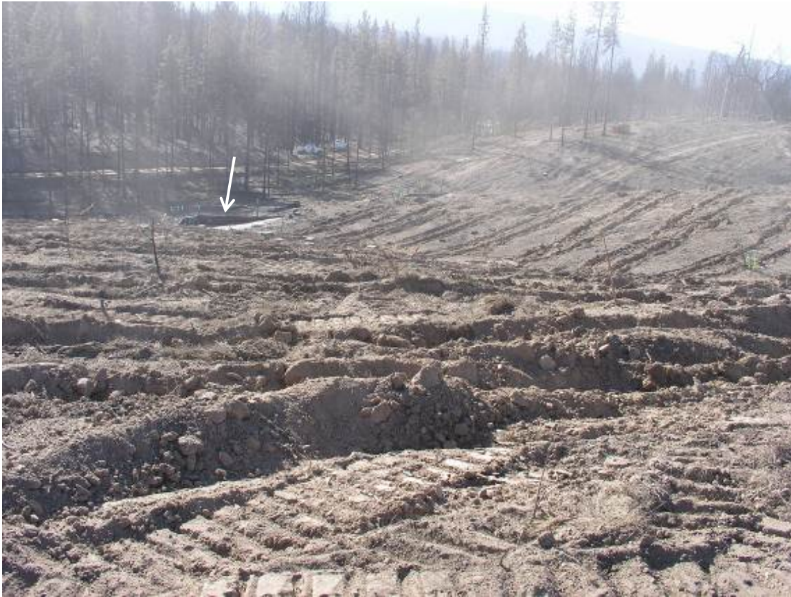
Figure ES-5. This photograph shows the downslope view from near the top of a swale treated with salvage logging plus biomass removal and contour subsoiling. The sediment fence is visible towards the upper left of the photograph (white arrow). The approximately 20-inch-deep furrows created by the subsoiling and the loose soil piled along their sides are evident throughout the swale. The furrows are oriented on contour with the slope or perpendicular to the downslope swale direction and interrupt water and sediment movement down the swale center. Note that the furrow orientation is not contour parallel on the contributing slopes. This combination of treatments produces the most site disturbance. Despite this visually stark and high level of disturbance, sites receiving these treatments produced substantially less water runoff and average soil erosion over the first winter season compared to the control sites (see Figures ES-7 and ES-8).
