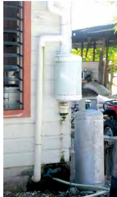
Water diverters installed by the PACC project.
