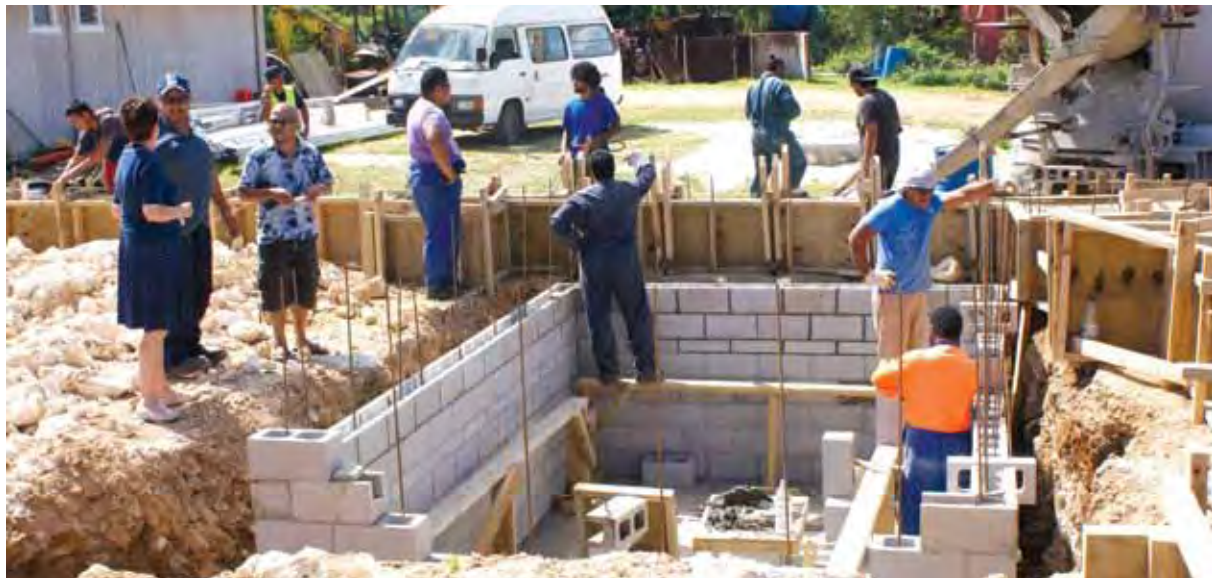
Top: Raising awareness at a sports day at Niue primary school. Bottom: The water tank moulding workshop under construction.
