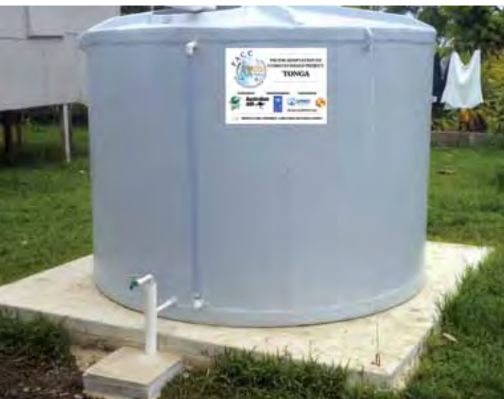
One of the 10,000 litre tanks.
