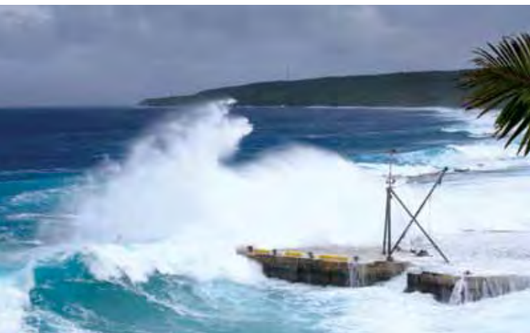
Heavy swells inundate the wharf on Niue. [Photo: Haden Talagi]
