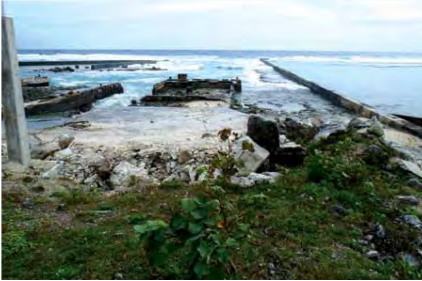
The harbour at Mangaia, Cook Islands, which was destroyed by cyclones in 2005.
