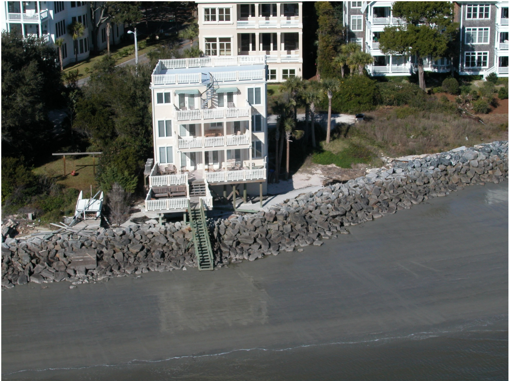
Ocean shoreline residence in high-risk eroding storm surge area, Saint Simons Island
