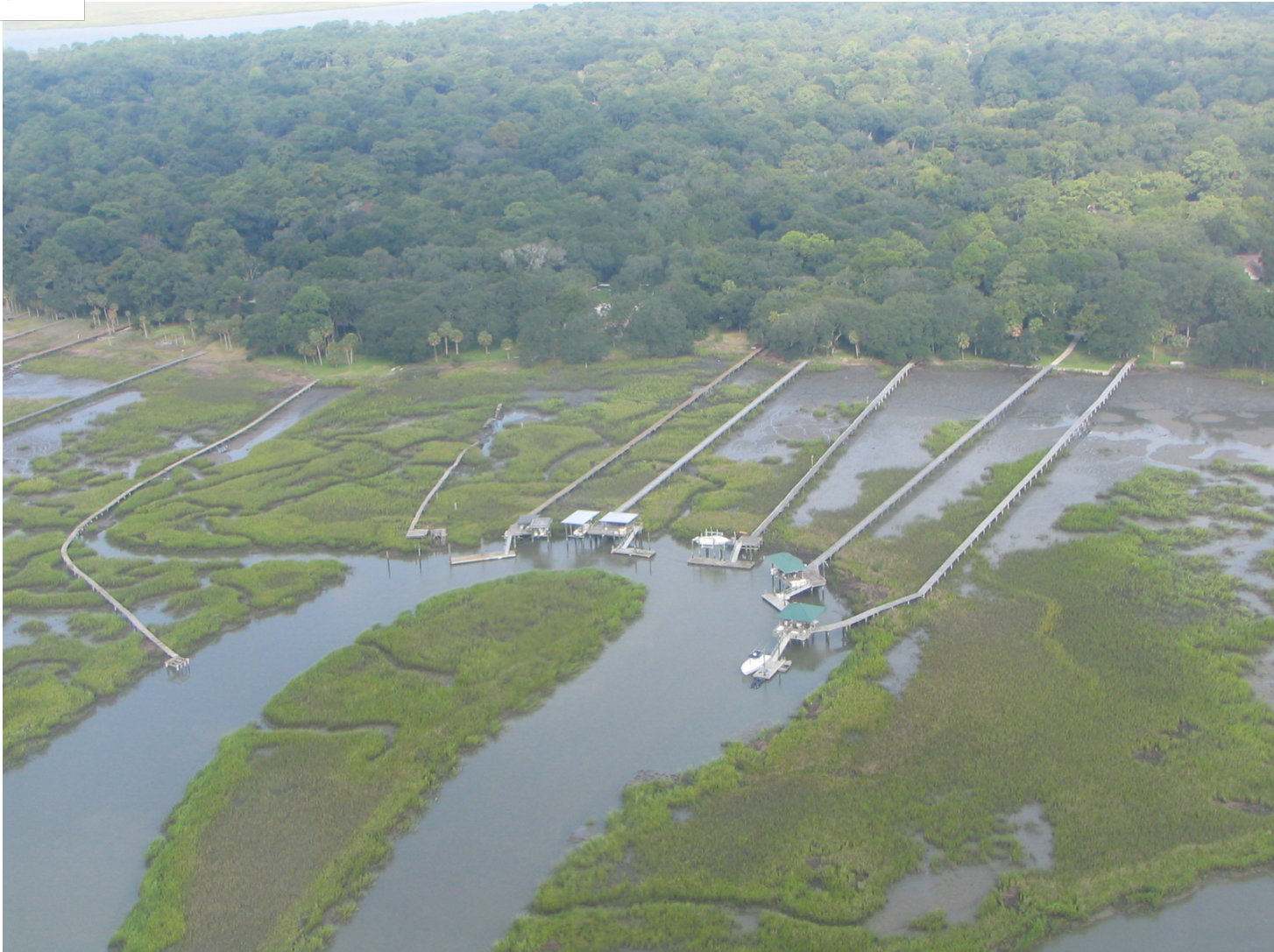
Long dock access across marsh
