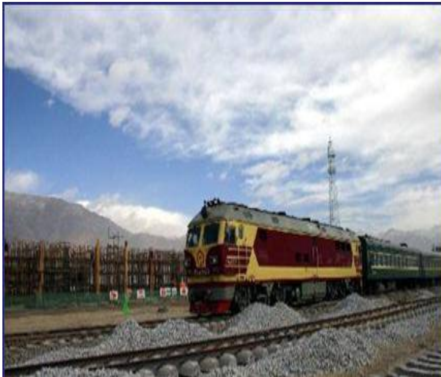
Qinghai-Tibet Railway Monitor and Control System
