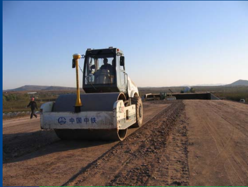
Railway 铁路: 智能压实
