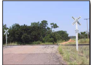
Figure 7.13 – A typical unguarded rail crossing, often found in rural areas. (Photo/Mike Wieder)
