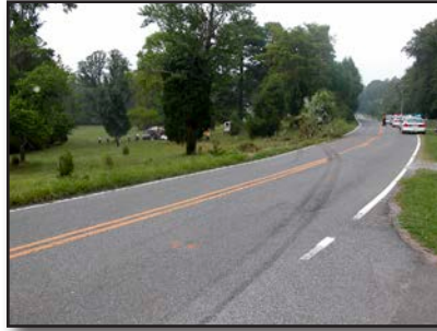
Figure 3.8 – The tire marks indicate the path of the vehicle after it was brought back to the road surface. (Photo/Robert Tutterow, Charlotte, North Carolina, Fire Department)
