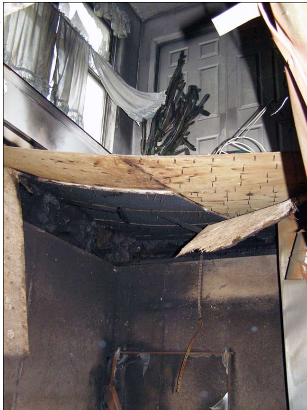
Photo courtesy of the Wea Township Volunteer Fire Department. Deputy Chief Steven Smith died when he fell into the basement of a residential structure fire.
