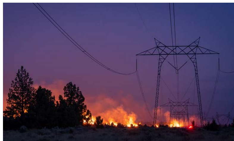
Wildfire burning under a high-voltage electrical transmission line. (iStock)
