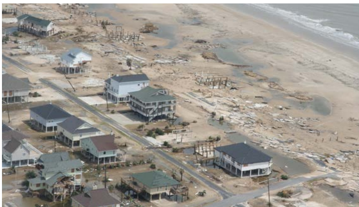
Storm surge damage caused by Hurricane Ike. Bolivar Peninsula, Texas, 2018. Photo courtesy of NOAA/Houston/Galveston National Weather Service Forecast Office; Houston Office of Emergency Management.
