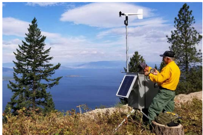
An Incident Remote Automatic Weather Station used on the Boulder 2700 Fire in Montana helped to provide real-time weather data for wildfire managers. Photo courtesy of Flathead Agency, BIA.
