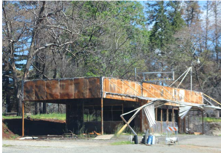
A burnt down business building after the Camp Fire in Paradise, California, in 2018. (iStock)
