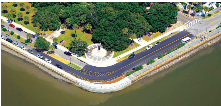
Aerial view of a sea wall in the City of Charleston.
