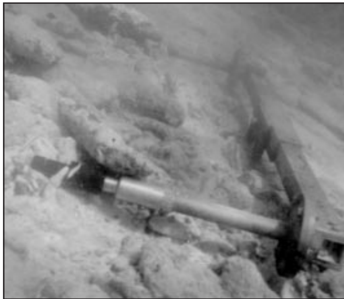
Fowey Rocks C-MAN cross arm and sensor mounts under 10 feet of water.
