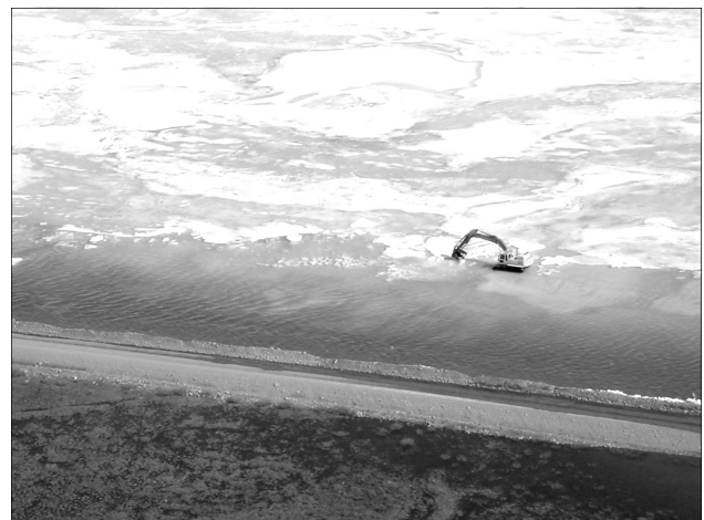
DOT frantically digs a channel in the overflow ice to keep spring runoff from the Dalton Hwy.
