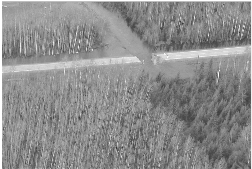
One of the three breaches DOT cut in order to relieve the flood waters.
