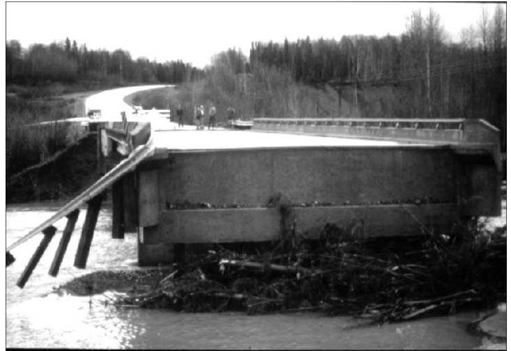
The approach to the bridge over Montana Creek on the Parks Highway washed out October 1986
