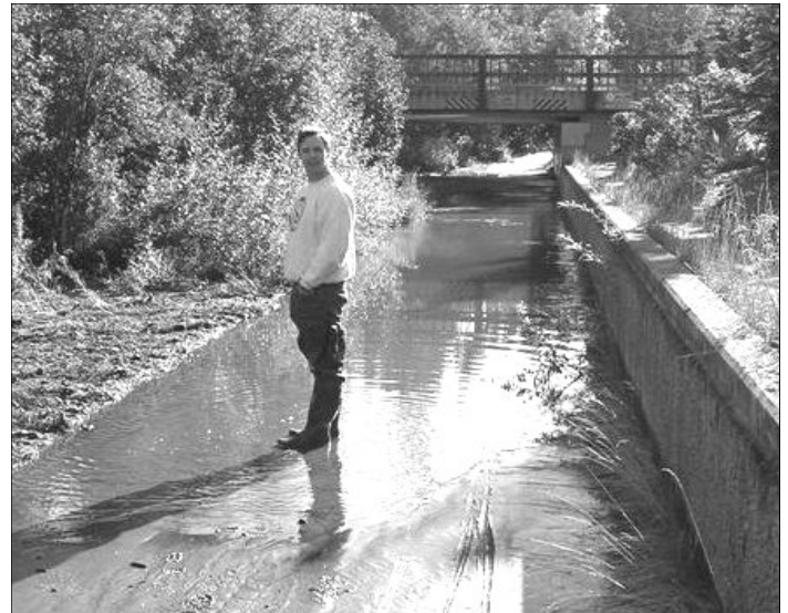
A few inches of water from Campbell Creek causes minor flooding of the bike path at Old Seward Hwy August 2006
