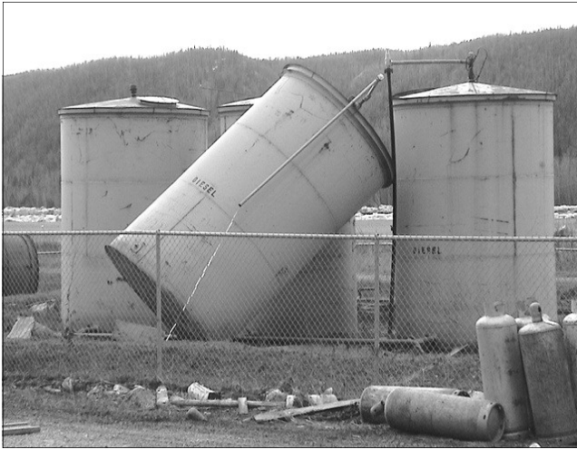
Fuel tank topples due to breakup related flooding in the village of Hughes on the Koyukuk River May 2003
