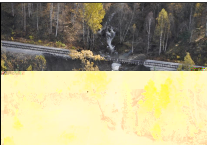
Flood waters from Gold Creek near the Susitna River leave railroad tracks hanging Photo courtesy of Alaska Railroad
