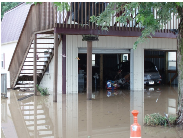
Flooding at Bagley, WI (July 2007)
