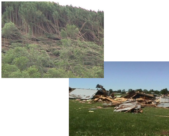
(Photos below: Thunderstorm wind damage in June 1998)
