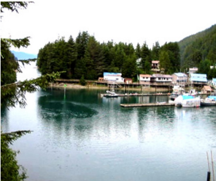
Elfin Cove from the wind tower of the inner cove with part of the “town” on the far shore.
