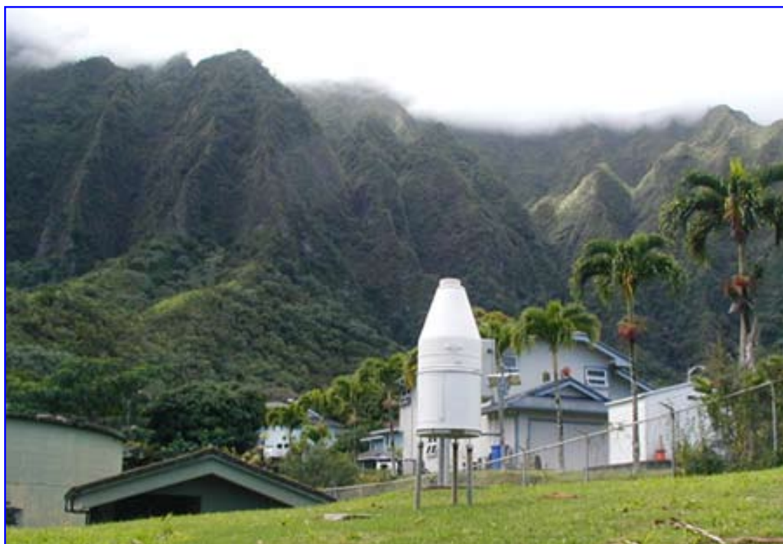
Electronic data loggers were installed to all 68 Fischer-Porter rain gauges in Hawaii, last summer. Pictured below is the Kaneohe, HI, site.
