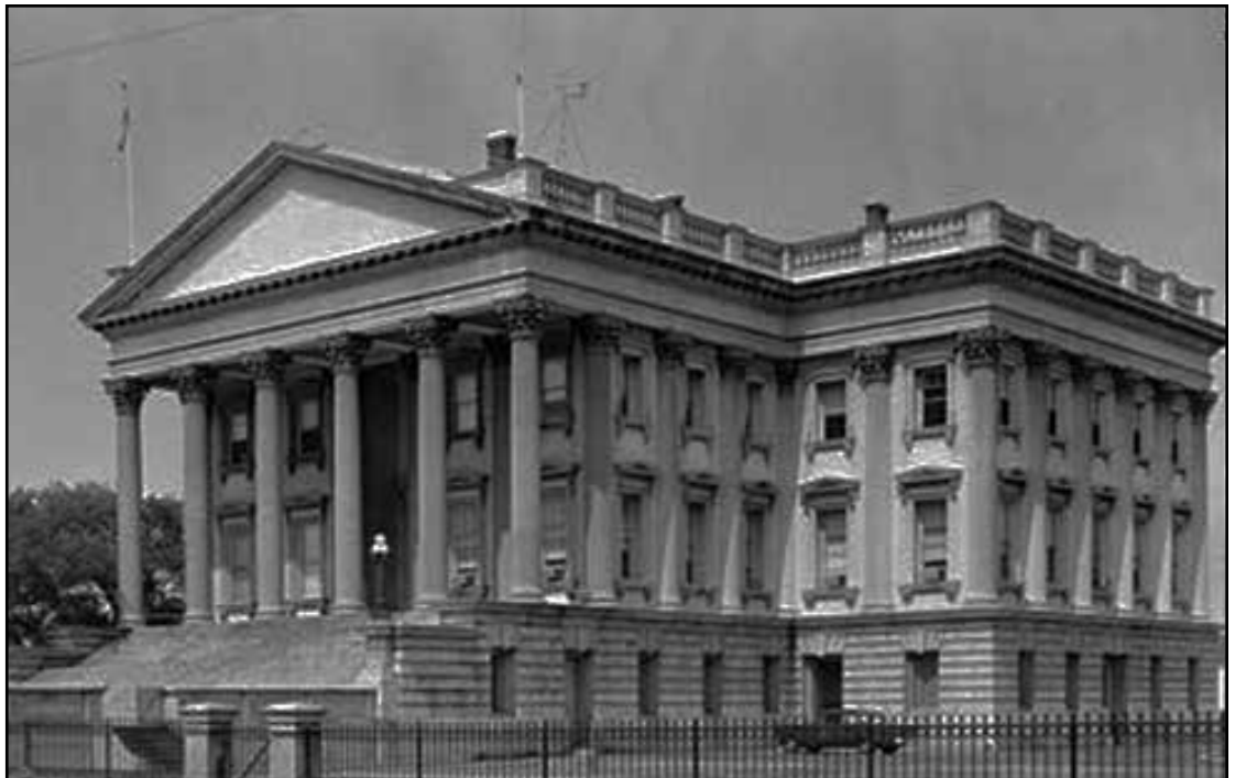
U.S. Customs House showing wind equipment on roof. Credit: Library of Congress.
