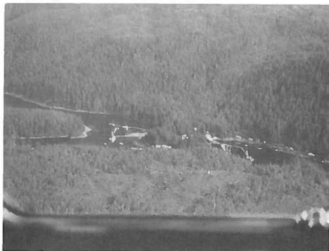
Aerial view of Elfin Cove looking east.
