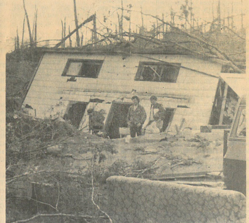
COOPERSTOWN — Mrs. Dorothy McCool, 48, of RD 1, Cooperstown, Venango County, was not home Friday evening when the tornado destroyed her home north of here. But when she returned home late that night and saw the structure, which had been blown off of its foundation, suffered a stroke according to her sons, who are pictured.
