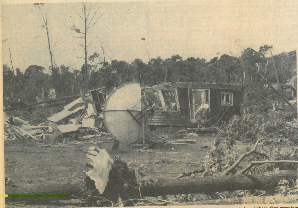
On Route 417 between Titusville and Franklin, half a TV satellite dish stands next to a house demolished by a tornado that tore
