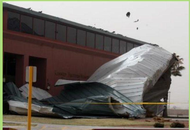
High winds near 50 mph damage a roof at the Kennedy Recreational Center in El Paso on March 16. (El Paso Times)
