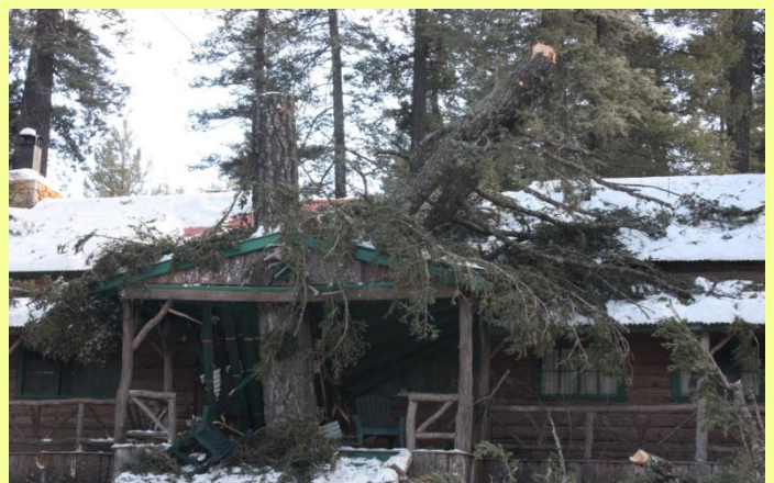
Wind damage at Cloudcroft NM. (John Fausett NWS/NOAA)
