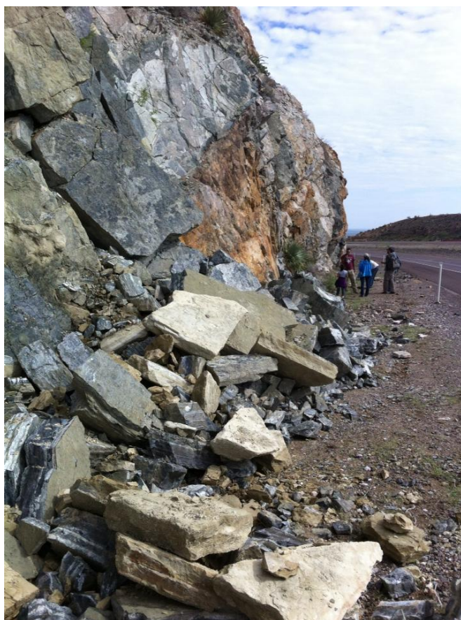
Heavy rains caused rockslides on Trans Mountain Road in El Paso. (Joshua Villalobos)
