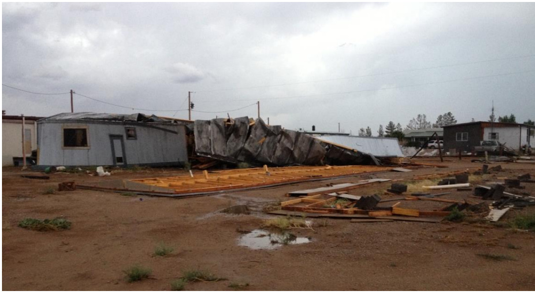
Thunderstorm winds of almost 90 mph destroyed buildings across Columbus NM on July 23. ( Mike Hardiman NWS)
