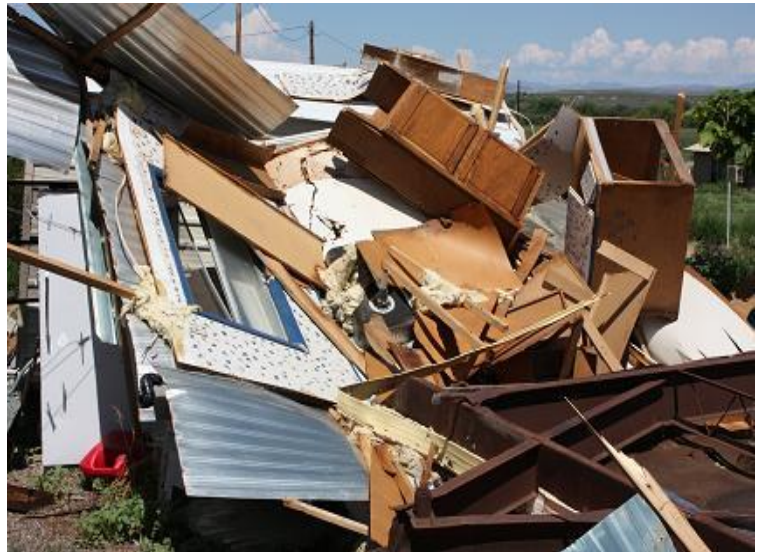
A thunderstorm microburst estimated at 90 mph destroyed this trailer home in Gila NM in 2010. (Mike Hardiman NWS )
