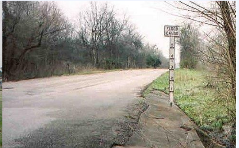
Flood gauge on Farm-to-Market Road 482, just south of New Braunfels
