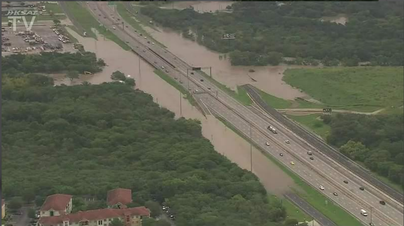
Figure 1: Flooding observed on July 6 th on US-90 at Leon Creek. Photo courtesy KSAT12 News.
