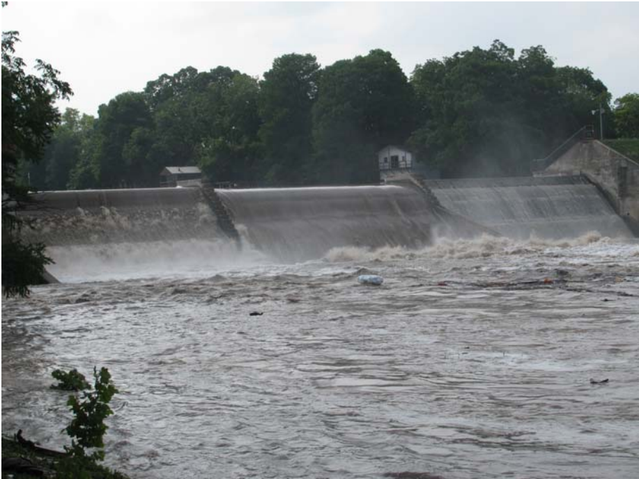
Photo 18, Dam on the Guadalupe at McQueeney
