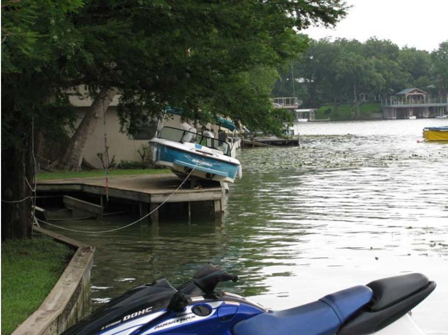
Photo 17, Many boats and homes were damaged on Treasure Island
