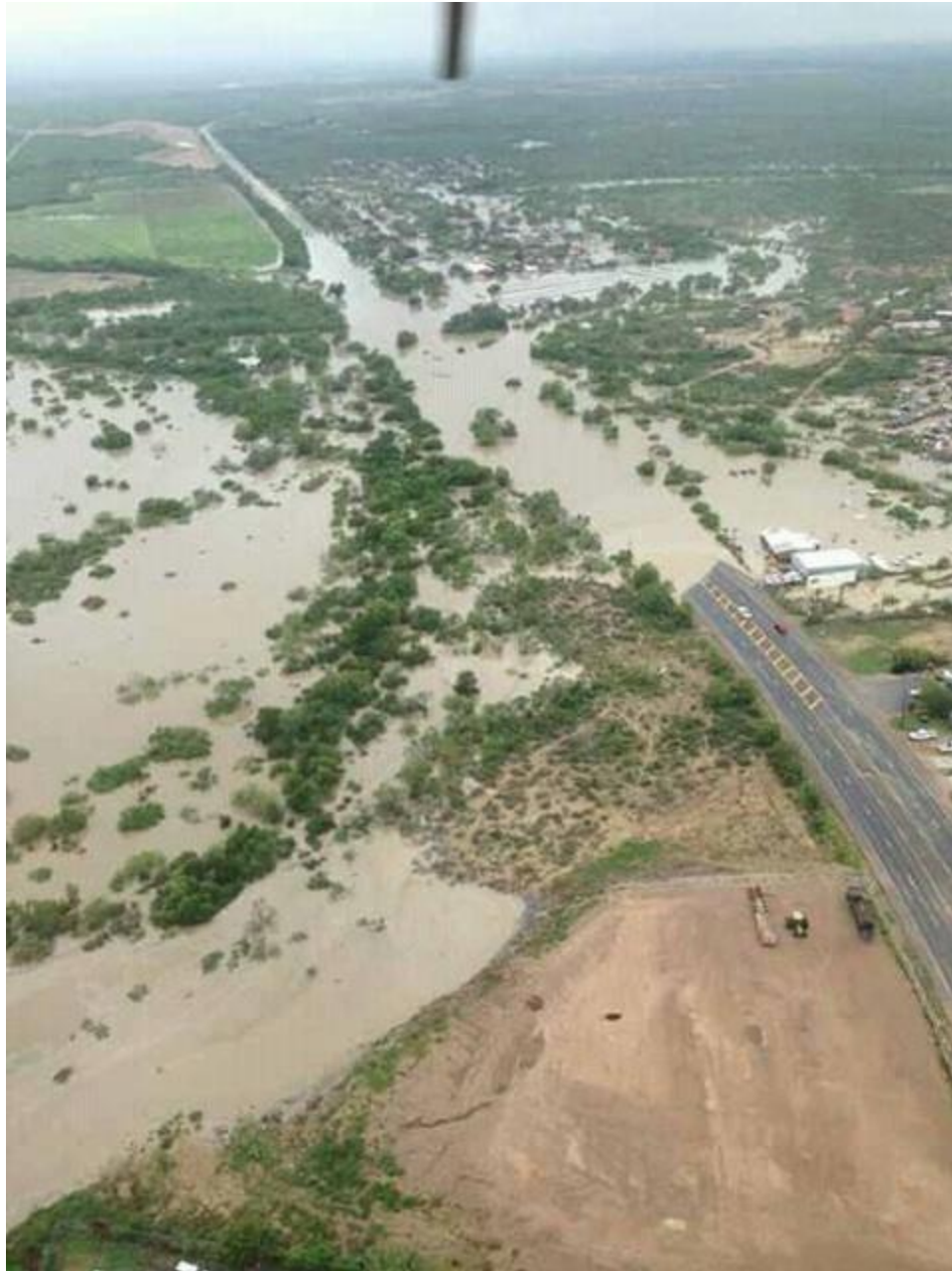
The photo above shows flooding along U.S. Highway 277 and Elm Creek. This photo is courtesy of the Eagle Pass Daily News.
