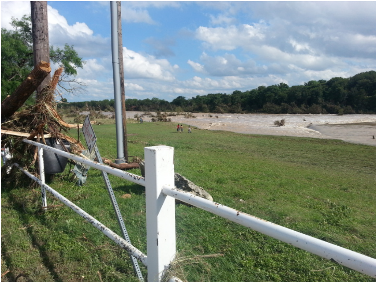
Blanco River Dam at Five Mile Dam Parks Complex in San Marcos, TX on May 24, 2015.
