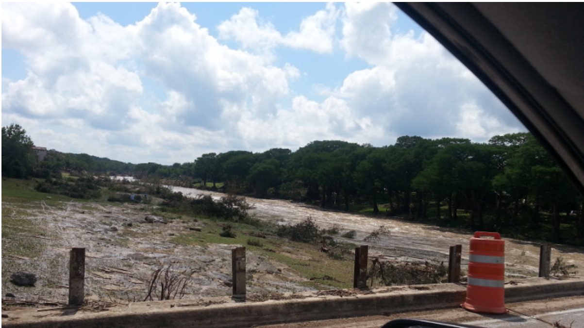
Upstream of Ranch Road 12 at Blanco River Crossing in Wimberley on May 24, 2015.
