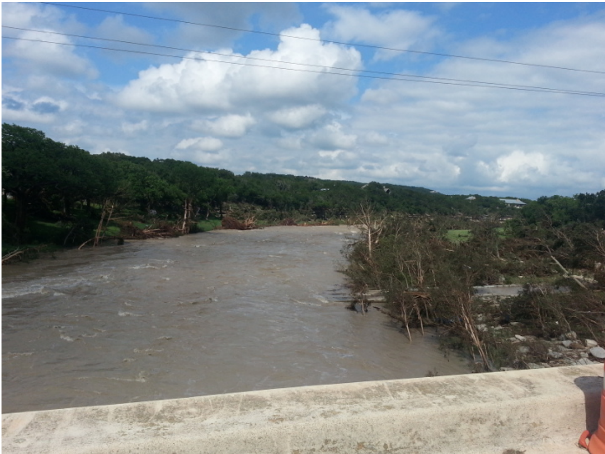
Downstream of Ranch Road 12 at Blanco River Crossing in Wimberley on May 24, 2015.
