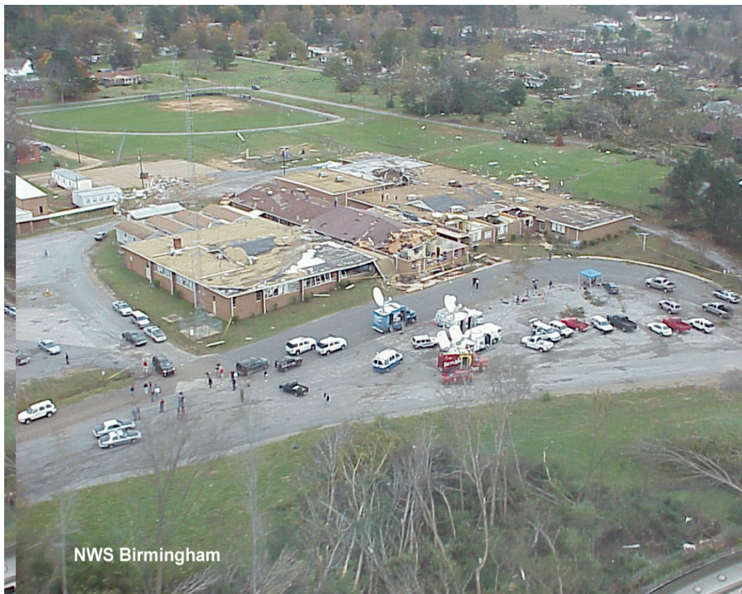
Carbon Hill Elementary School, Carbon Hill, Alabama, after being struck by an F3 tornado on November 10, 2002. (NOAA)
