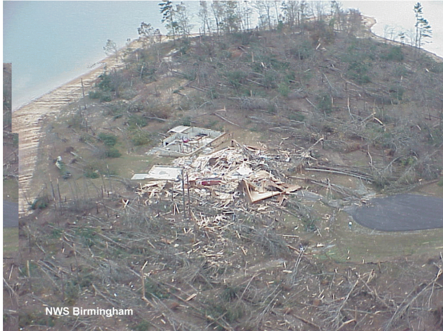
Destroyed house from an F3 tornado in Winston County, Alabama, on Smith Lake, about 5 miles southwest of Arley. This was from the path of the Carbon Hill tornado that crossed three Alabama counties—Fayette, Walker, and Winston—on November 10, 2002. (NOAA)
