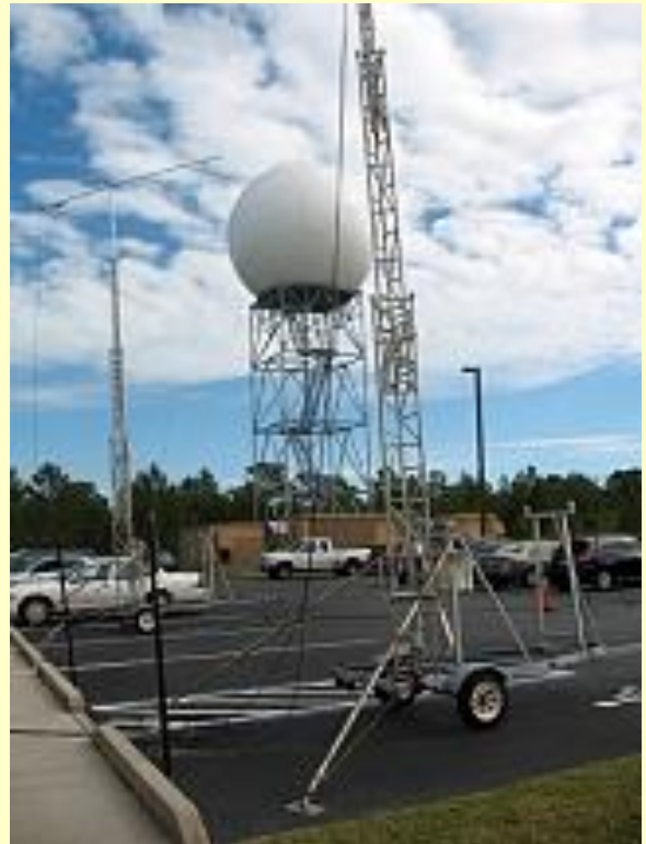
Portable VHF towers with 2m & 6m VHF beams
