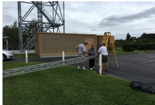
Getting the PCARS tower ready to raise the A-4S beam
