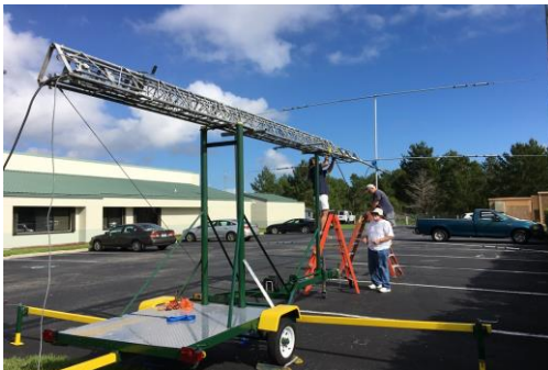
Setting up the A-3S beam on the MCARA tower
