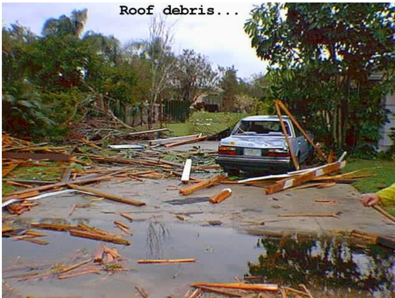
Damage photo at location 2.
