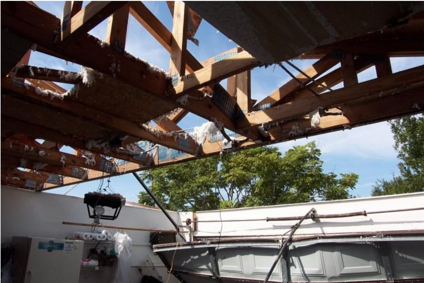
Removed section of roof (inside view).
