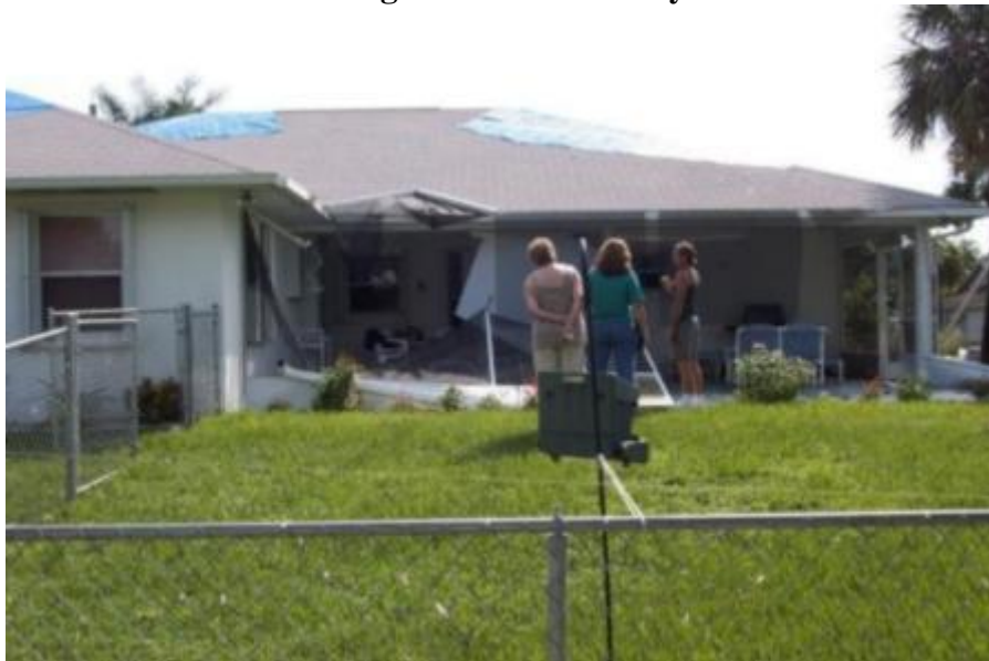
Demolished screen house of nearby home.
