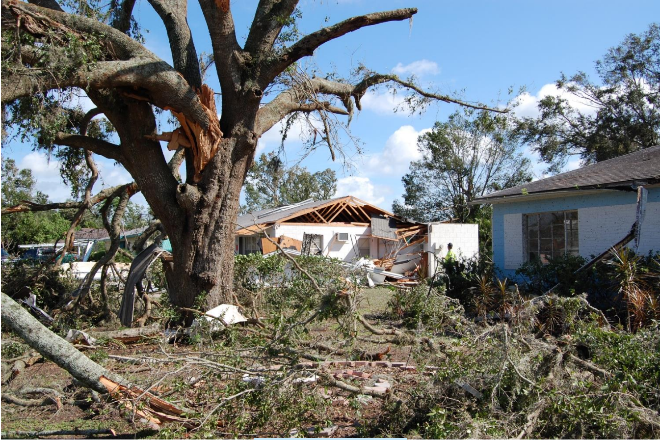
EF-1 Damage to Home
