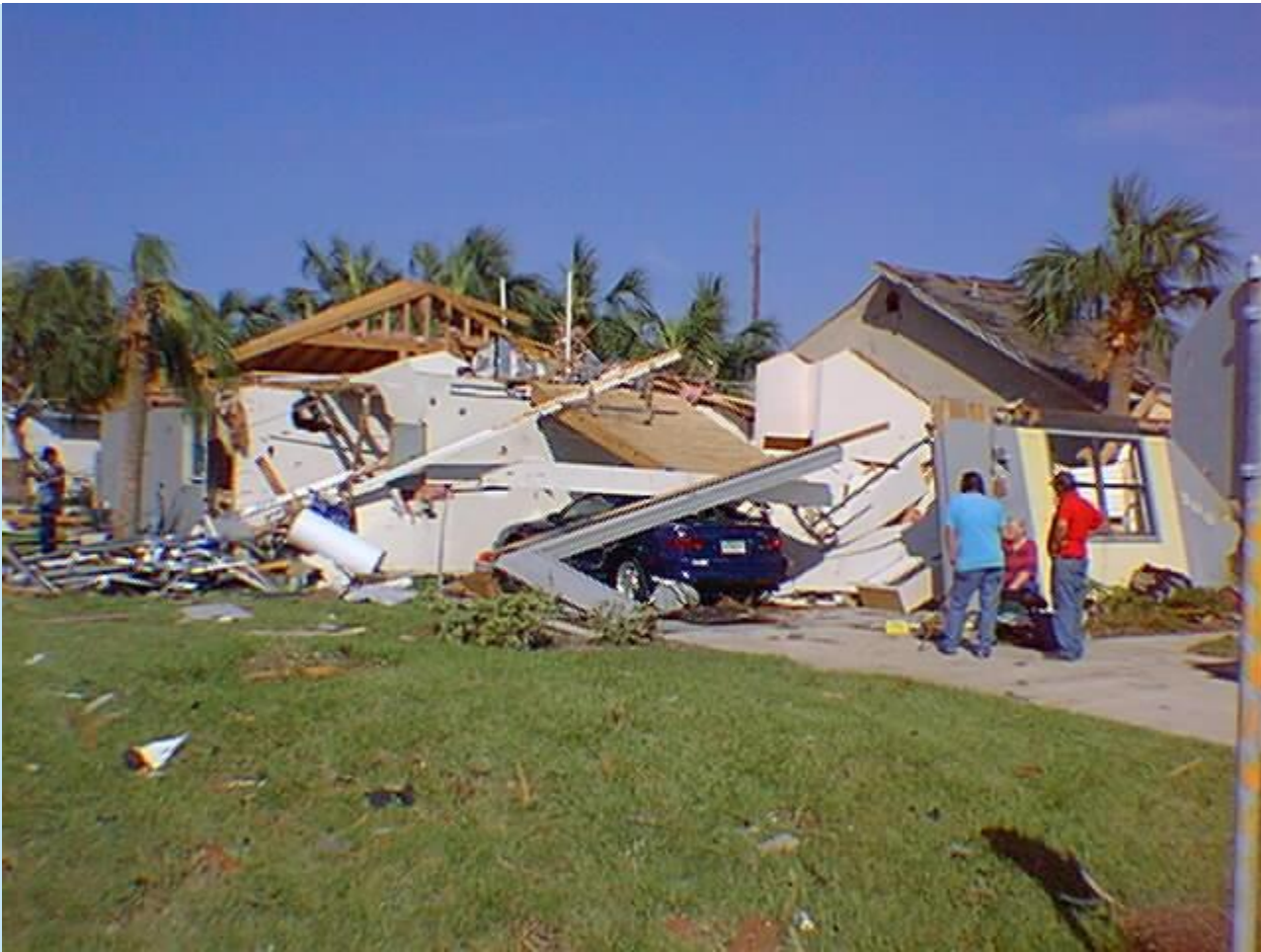
Location 6. Severe damage to a home.
