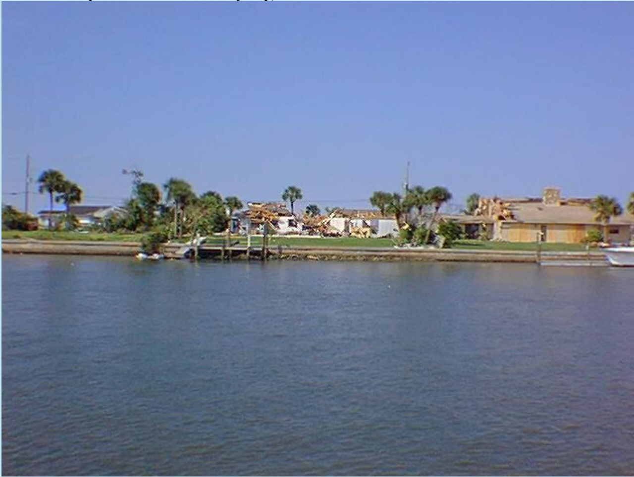
Location 1. Damage to canal
