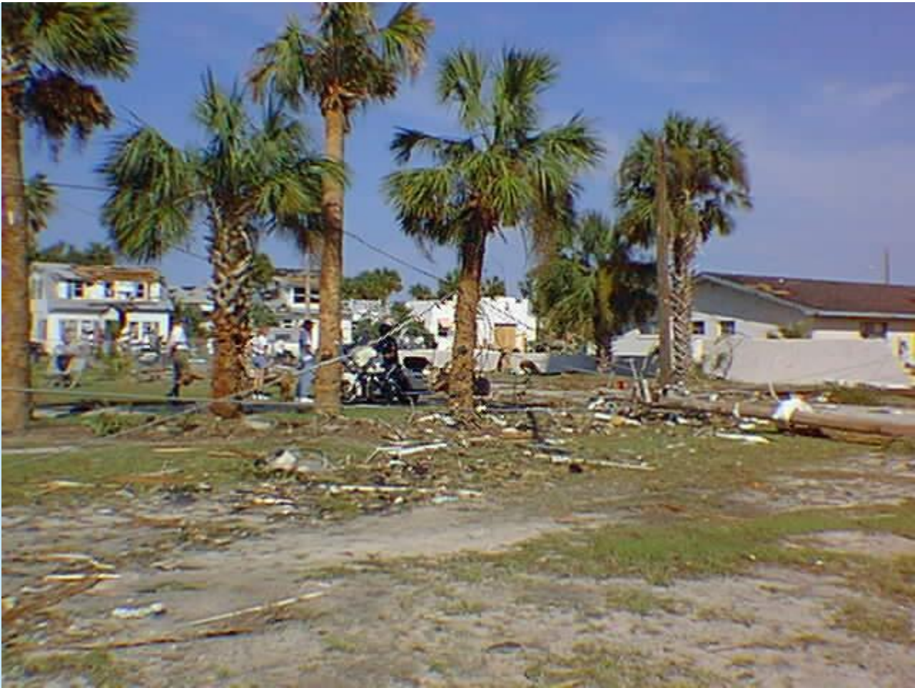
Location 3. Debris field.
