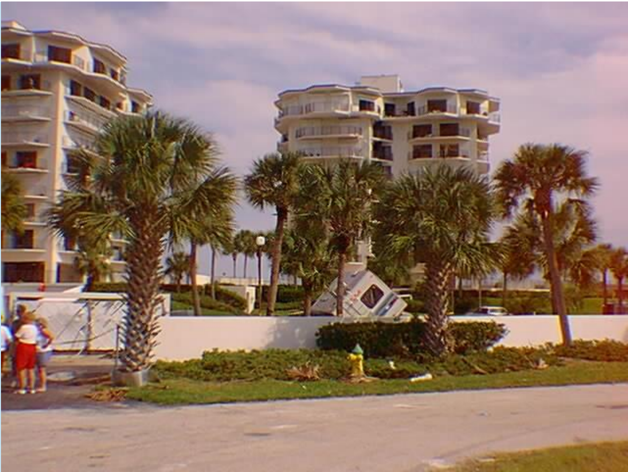
Location 2. Damaged Condo.
