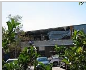
F0 damage to warehouse in Seminole County
