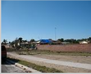
Path through a brick wall in Seminole County.
