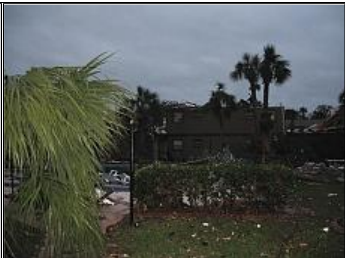
Damage to Apartments in Daytona Beach
