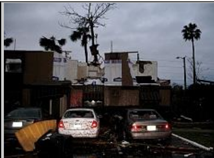
Damage to Apartments in Daytona Beach
