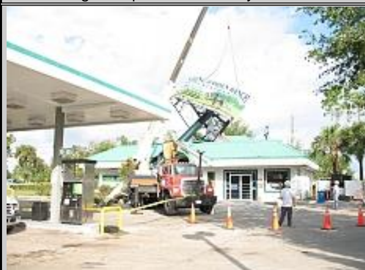
Damage in the Deland Area
