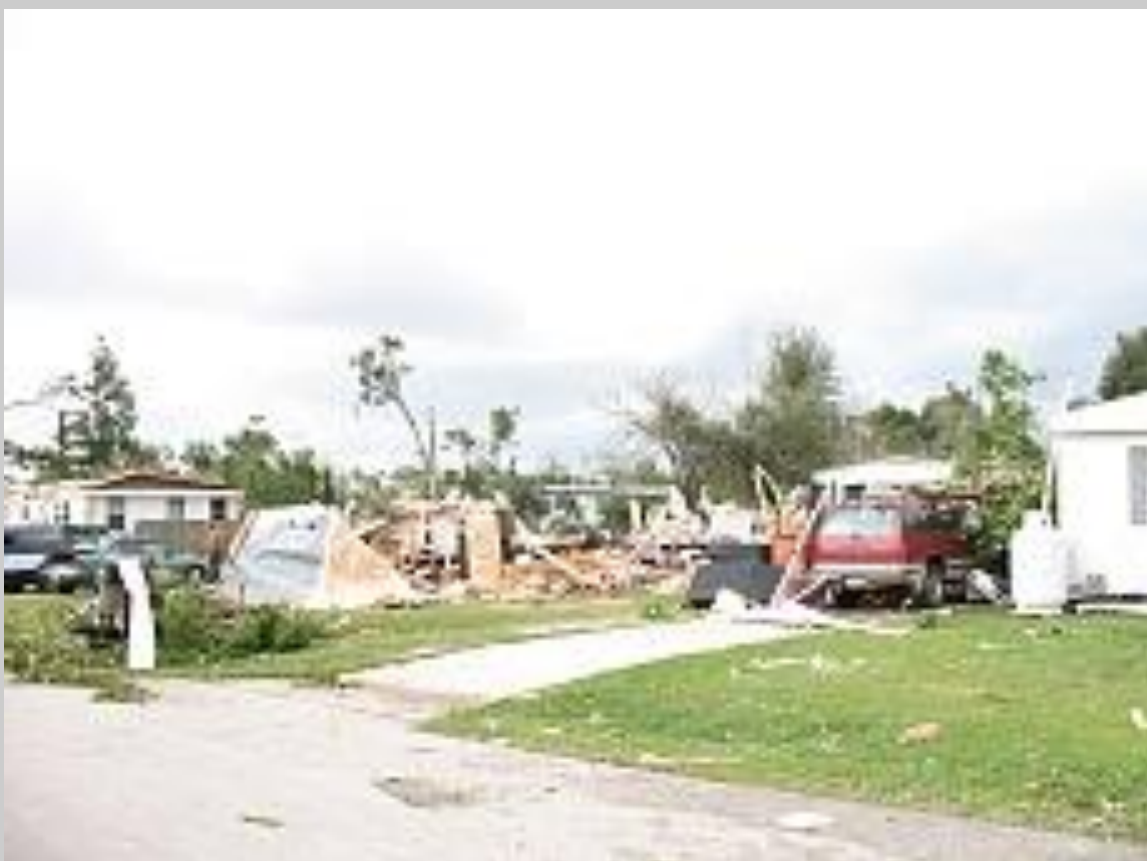
Damage in the Deland Area
