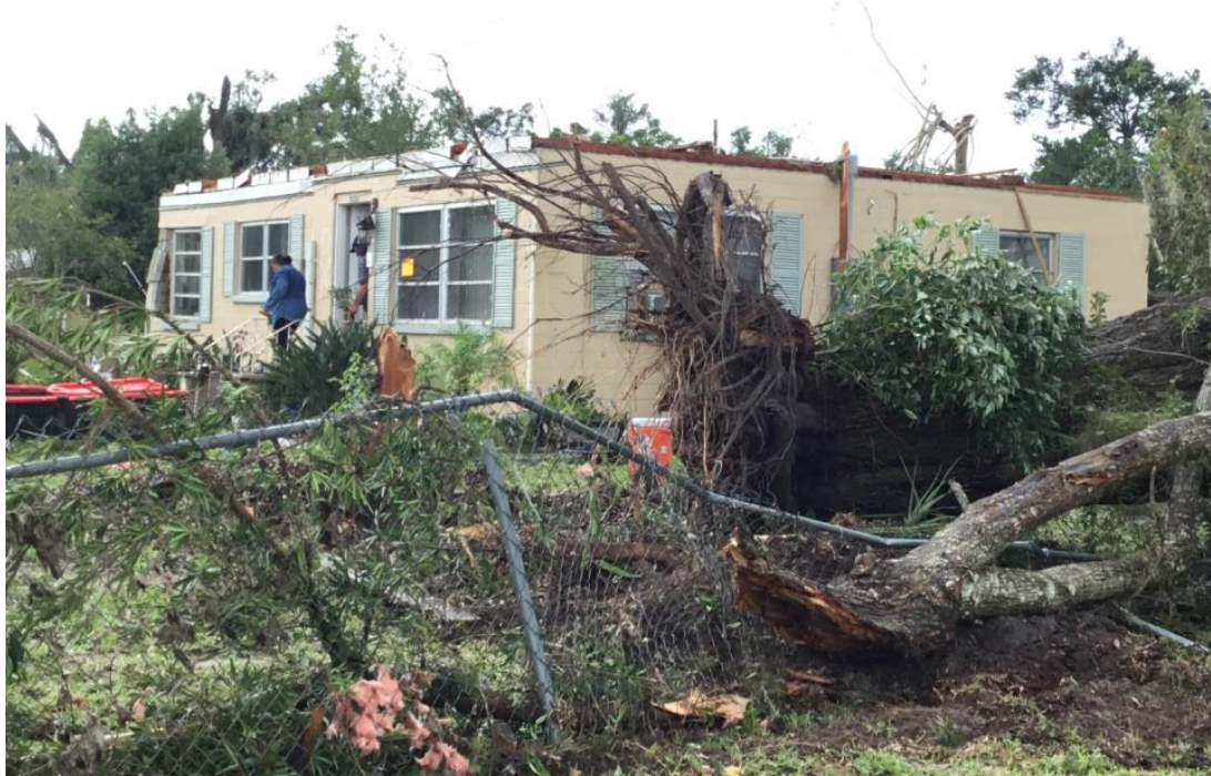
EF-2 tornado damage to homes along E Washington Ave.
