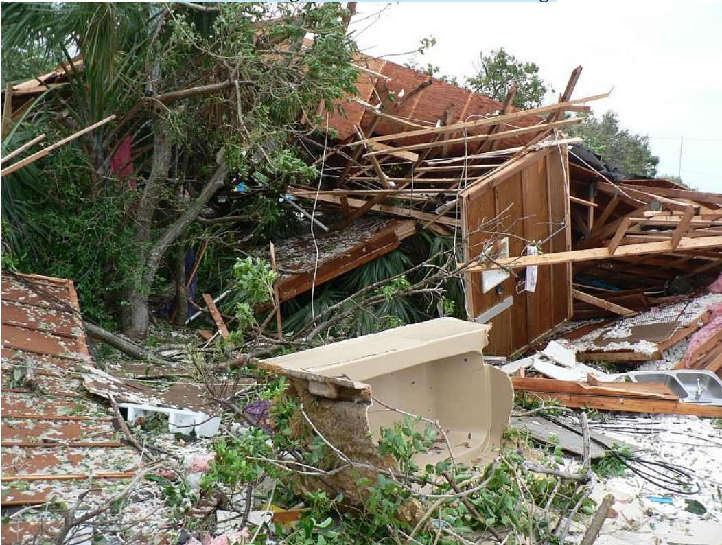
Tornado Damage North of Sebastian Inlet Bridge
